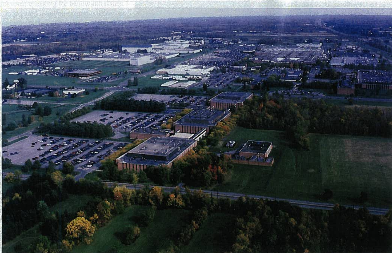
Photo 1: Xerox was able to increase efficiency and interoperability, as well as reduce costs, at its Webster, N.Y., campus by implementing a BACnet-based system. The campus includes research, engineering and manufacturing areas, cafeterias, offices, and conference rooms.
